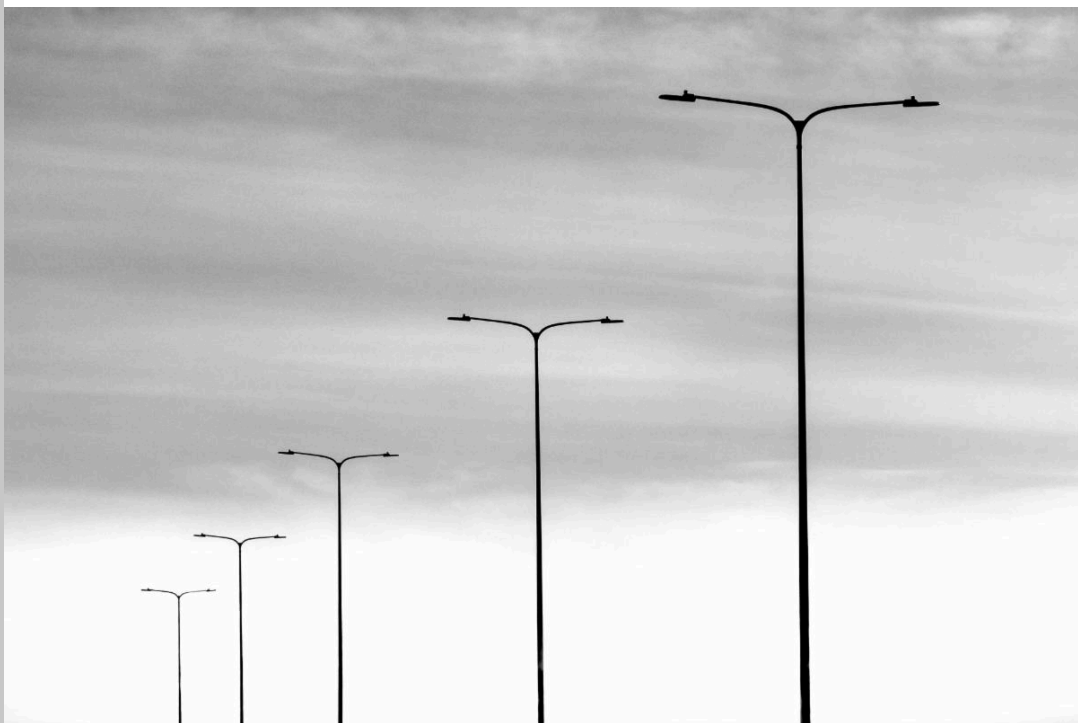
Light Poles No. 22
